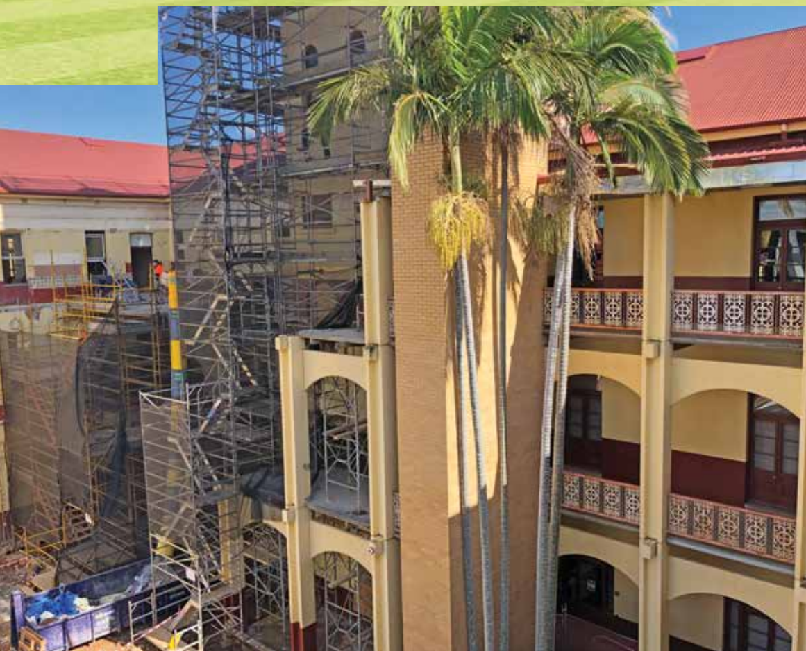
Treacy precinct construction.
